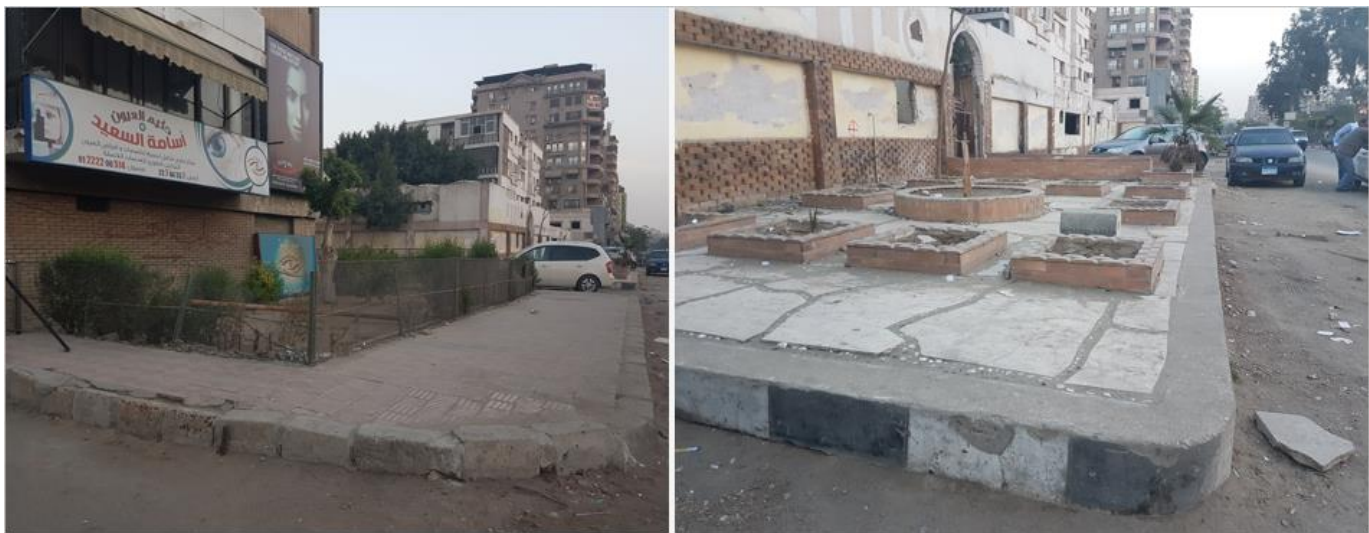
Photos (17) Different types of encroachments on the pavement
